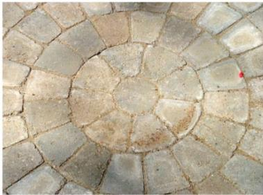
Manufactured Pavers come in many sizes, including a special mix that creates a radius pattern like this one.
